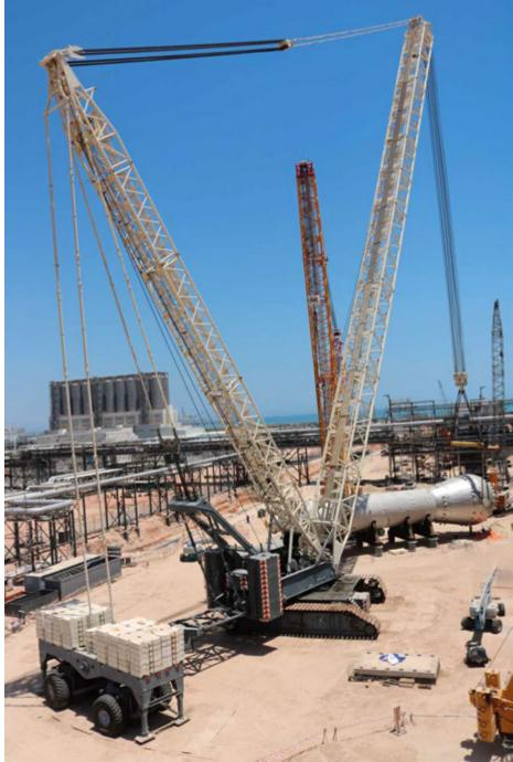
The reactor was lifted with the 1,600 tonne crane rigged in 'Superlift' configuration and then transported to its installation area. AJHL's unique ability for exceptional planning enabled the precise lifting of the reactor in a confined space while maintaining minimal site disruption. The project's outstanding achievement was not merely its timely completion but its meticulous orchestration, which defines AJHL as a true market leader.
