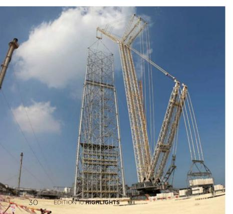
demountable flares during the upgrading of the largest refinery in Saudi Arabia, located in the Eastern Province. With an assembly derrick height of over 200m and the heaviest preassembled top module exceeding 160 tonnes, the heavy lifting job was executed by using a highcapacity 3200 tonne crawler crane with a twin boom attachment.
