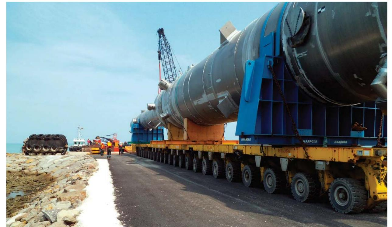
this setback AJHL's engineers proposed an alternative methodology to shift, barge and deliver the heavy equipment from storage to the project site. A carefully-scheduled SPMT delivery phase using 2 PPU and 28 axle lines ensured the equipment was delivered directly under the hook of the cranes and timed to co-ordinate with the planned lifts of all the equipment. The next phase saw the Demag CC2800-1 built into 108m SSL-LSL configuration and travel to the new flare.
